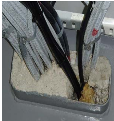
Sealing not done using fire retardant material
