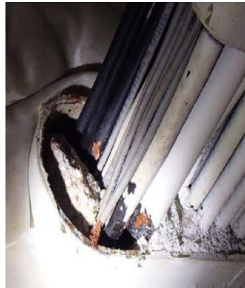
Sealing not done using fire retardant material
