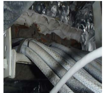
Sealing not done using fire retardant material
