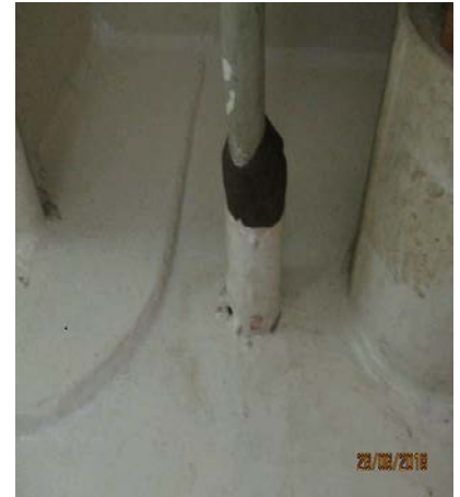
Fire retardant compound inserted on pump room cable penetration
