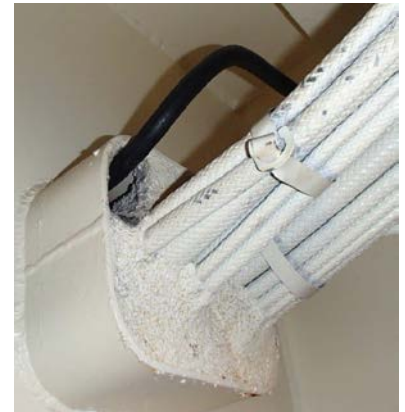
Sealing not done using fire retardant material
