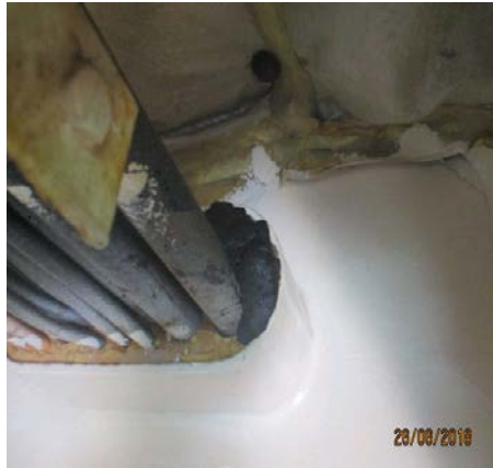
Fire retardant compound inserted on carpenter store cable penetration
