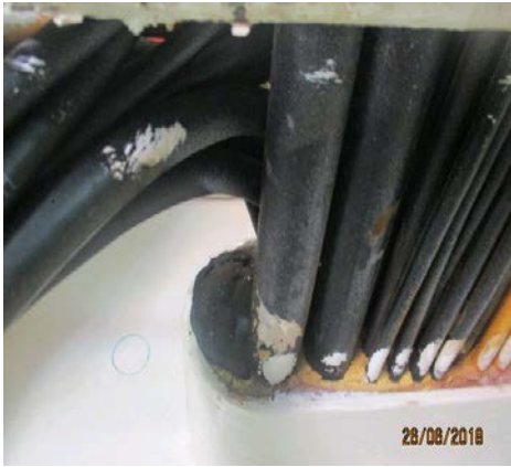
Fire retardant compound inserted on bosun store cable penetration
